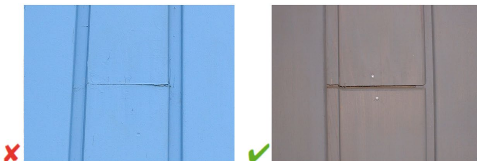
Figure 8 - Butt joints incorrectly installed (Source: Centrum Hout, 2024)
